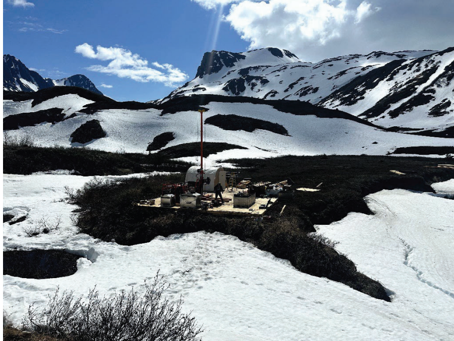
Tunnel Boring Alignment Drilling Platform
