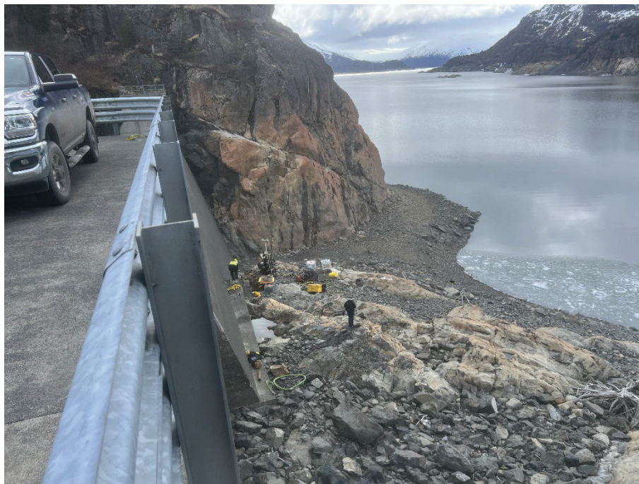
Frontside of Spillway Drilling
